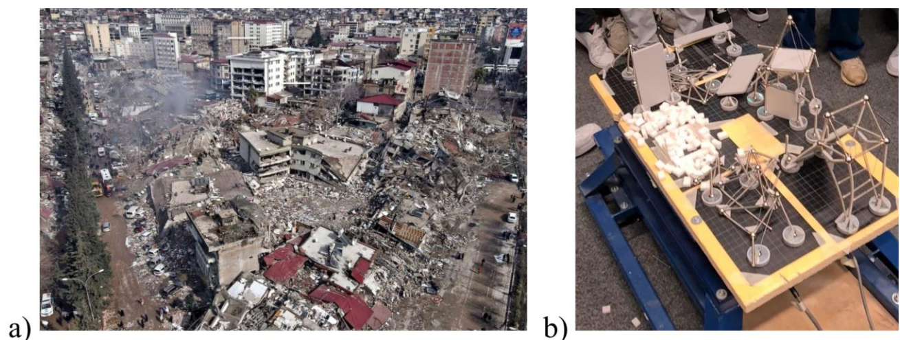
Figure 1 : Regional response to earthquake load: a) destruction in the urban center following the 2023 Kahramanmaras, Turkey earthquake (Abraham et al. 2023), b) demonstration of the city-scale response using the activity kit models and a small-scale shake table.
